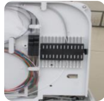
2. Connect small diameter cable with splitter input cable by fusion splicing or mechanical splicing
